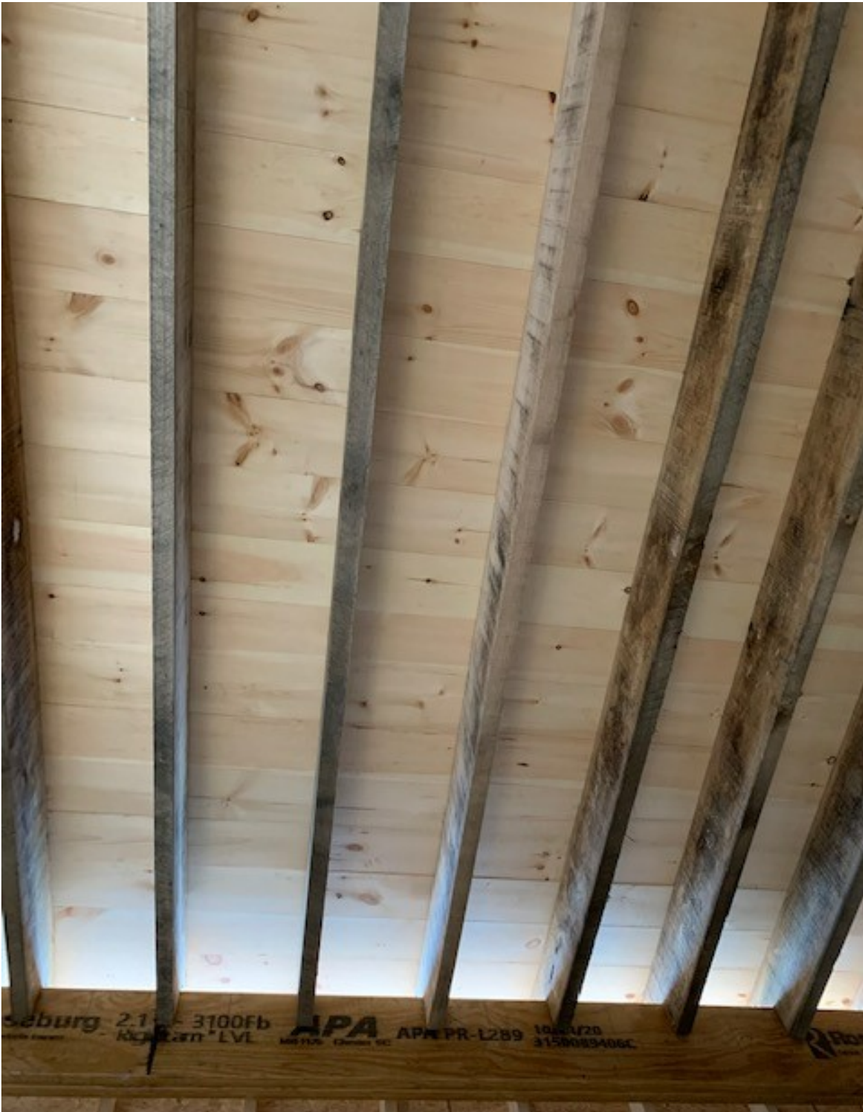
Pictures of new roof: 2 LVLs, rough cut rafters, and pine slats
