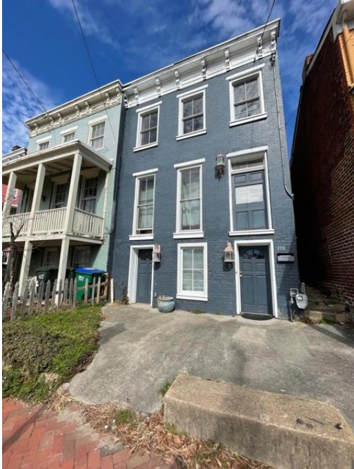
Figure 1. Front façade, 116 W. Leigh St.
