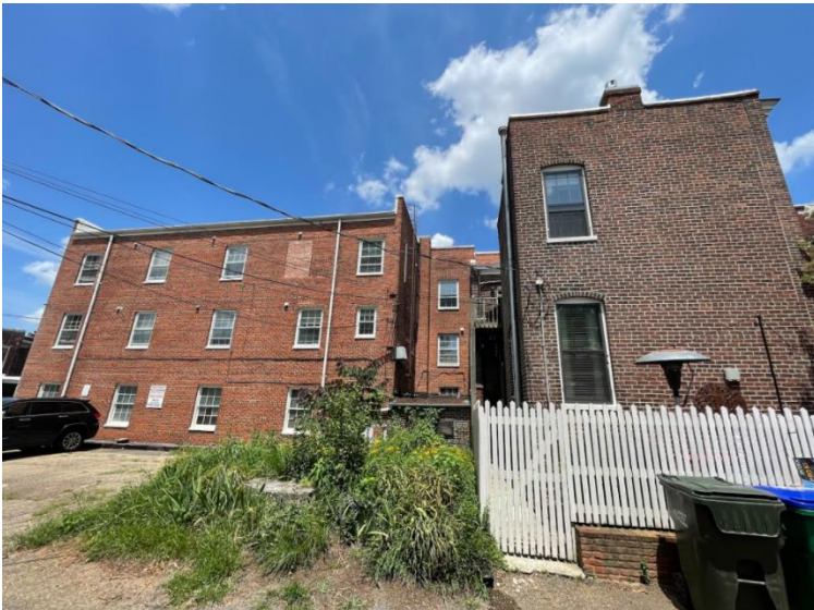
Figure 5. View of existing 2 nd story deck from the alley
