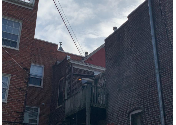
Figure 4. Roof visibility from the alley.
