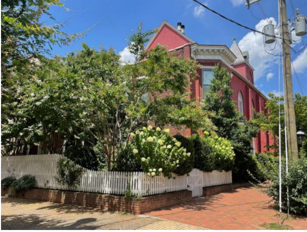
Figure 7. View of side of property from N. 26 th
