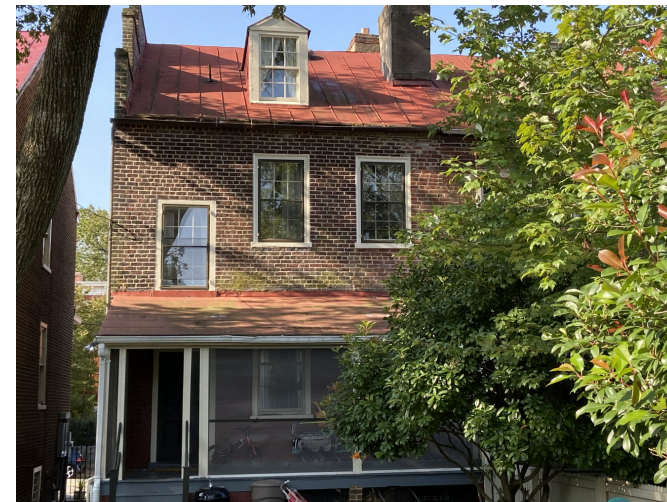
EXISTING REAR PORCH
