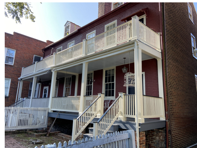
NEIGHBORING REAR PORCH
