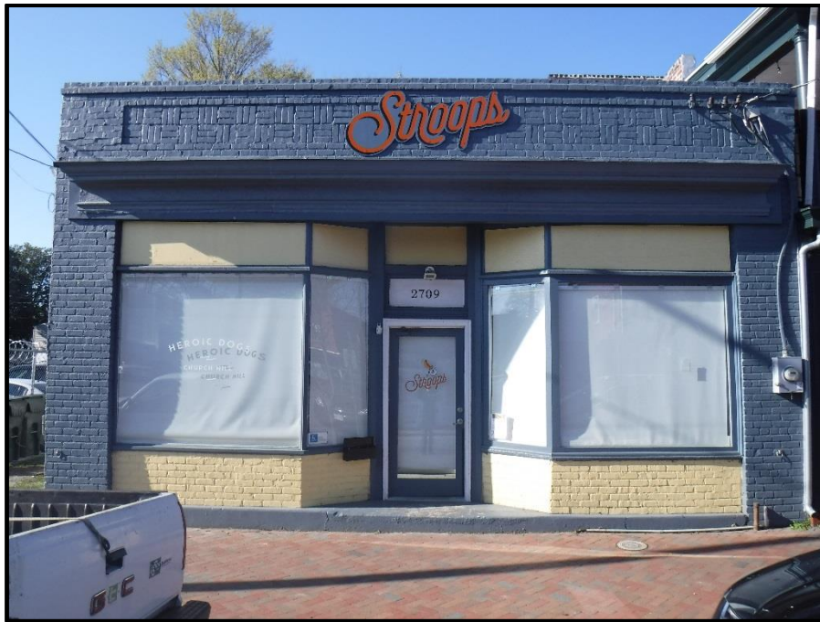
2709 East Marshall Street (March 2018)
