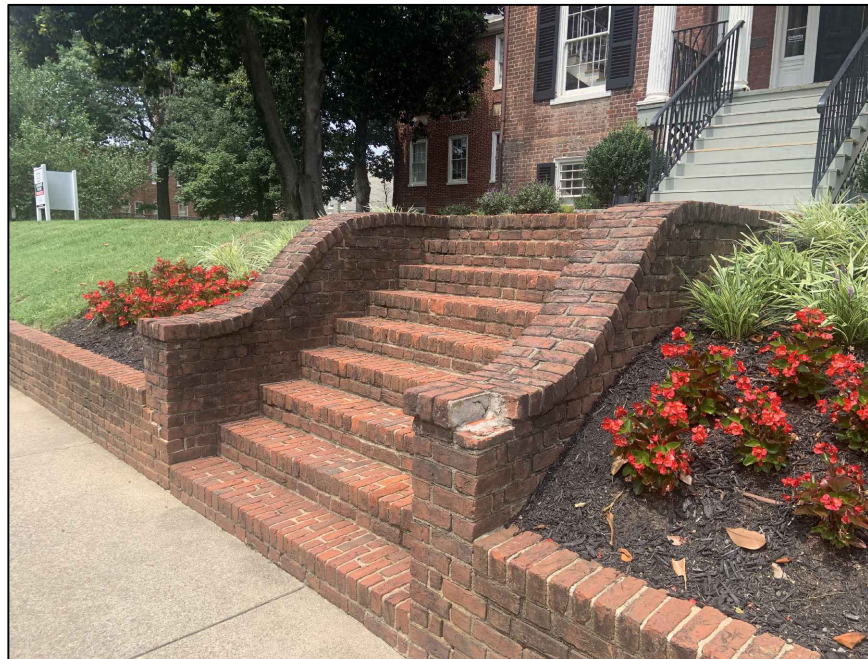
EXISTING STAIR NTS
