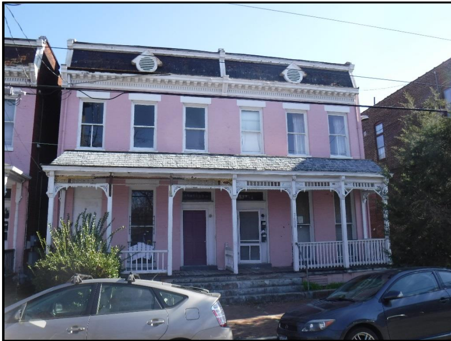
2406-2408 East Clay Street (March 2018)
