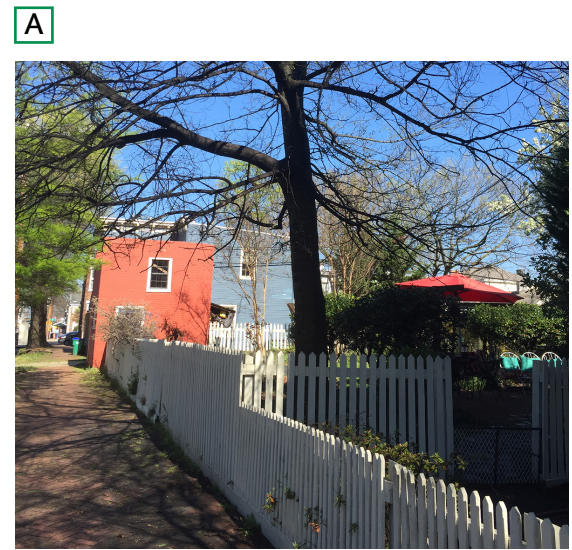
Photo A illustrates existing carriage house elevation (M St. sidewalk view)
