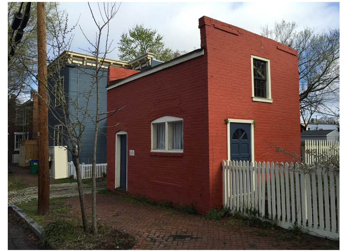
Photo A illustrates existing carriage house elevation (M St. sidewalk view)
