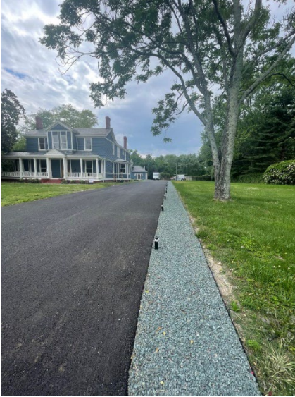
Figure 1. 4002 Hermitage, 2023. View looking west along driveway and side yard.
