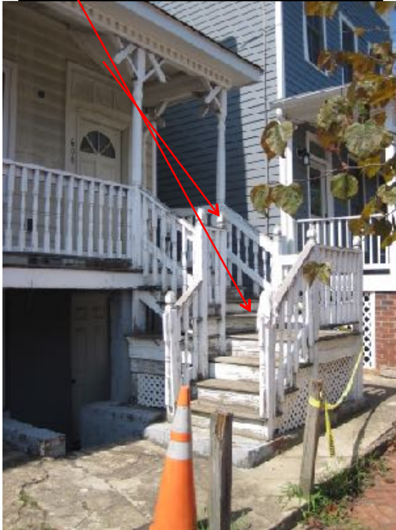
Current stairs and railing
