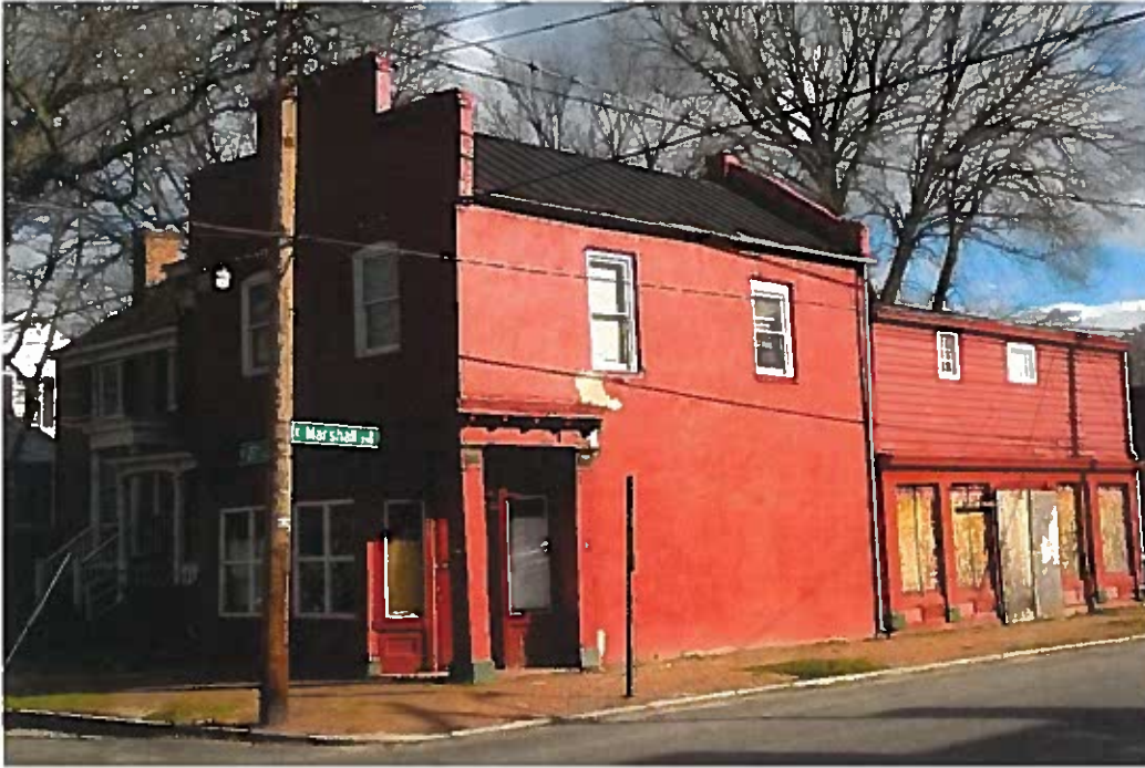
CURRENT BUILDING CONDITIONS
