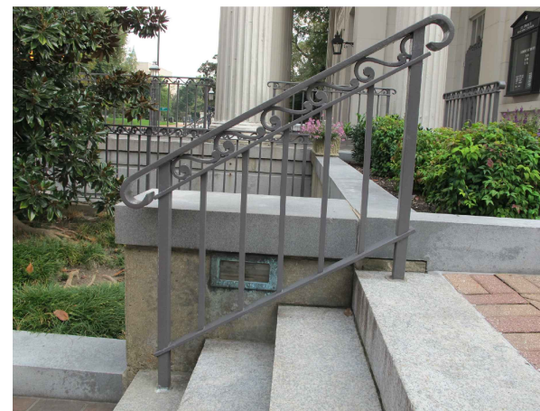
3 Photo of Existing Railing Not To Scale
