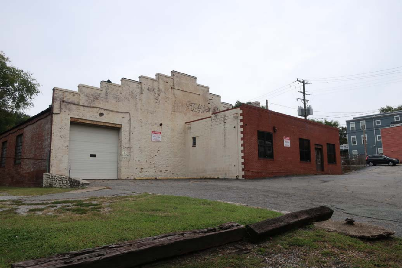
1. Historic garage at 21st and Broad
