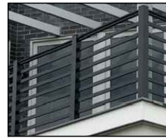
METAL GUARD HORIZONTAL INFILL, DARK BRONZE OR BLACK FINISH
