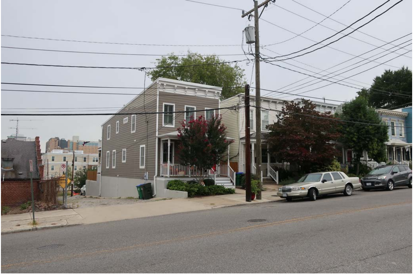
8. Existing houses on south side of 21st Street
