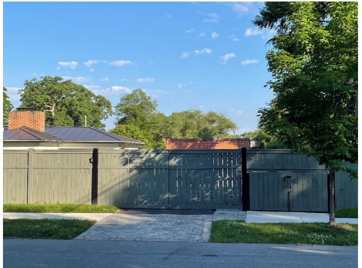
Figure 2. View of the southeast elevation of the garage, which is obscured behind a wooden fence.
