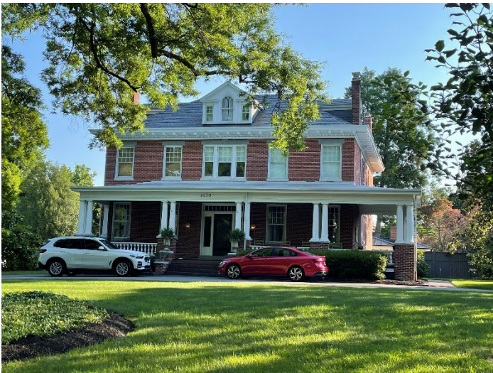
Figure 1. View of the façade of 1630 Pope Avenue, which faces Hermitage Road.
