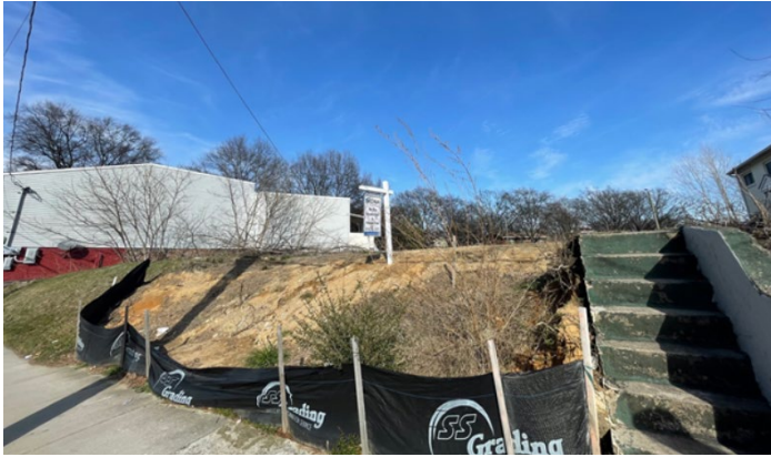
Figure 3. View from Mosby Street
