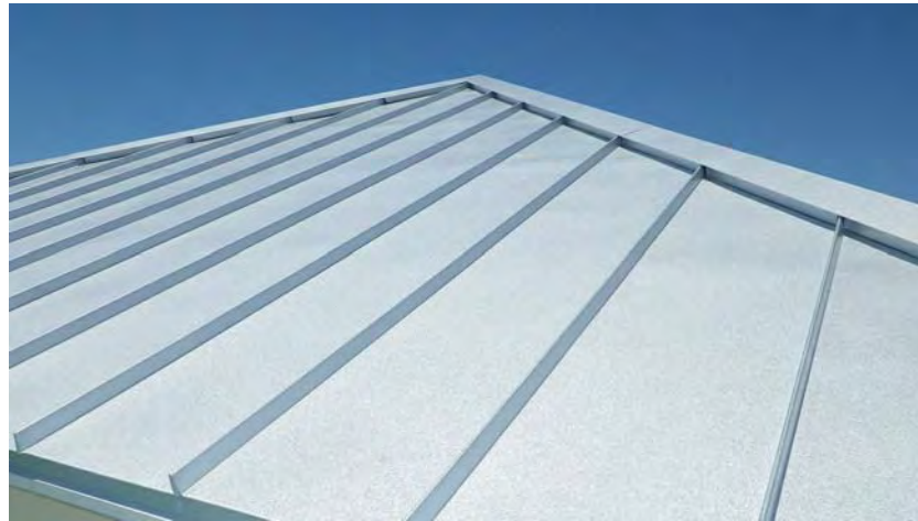
ROOF: METAL STANDING SEAM
