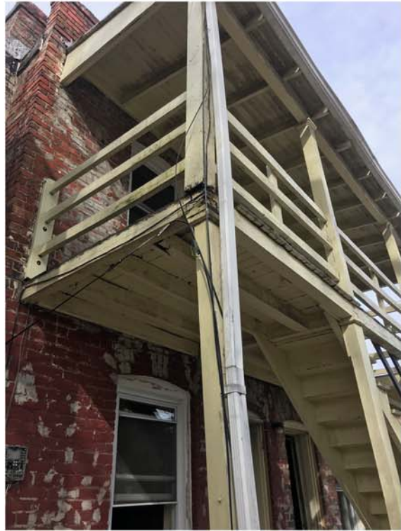
CURRENT PHOTOS OF BACK PORCH FAILING POSTS
