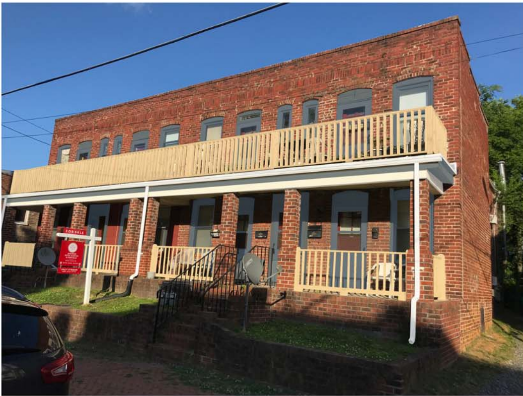
PROPOSED PHOTO OF FRONT RAILINGS PAINTED TO MATCH EXISTING & WOOD TRIM TO MATCH REAR DECKING
