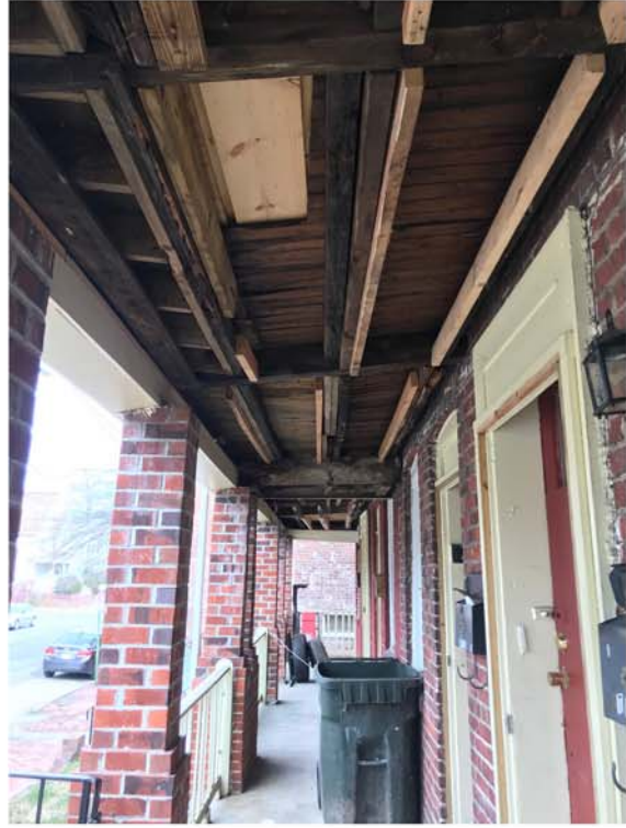
CURRENT PHOTO OF FRONT 1ST FLOOR CEILING FRAMING
