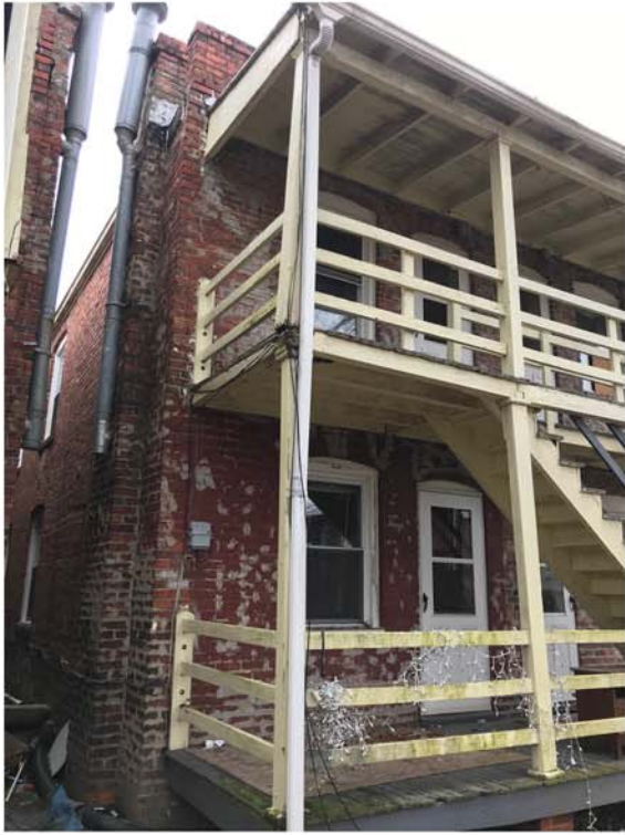
CURRENT PHOTOS OF BACK PORCH FAILING POSTS
