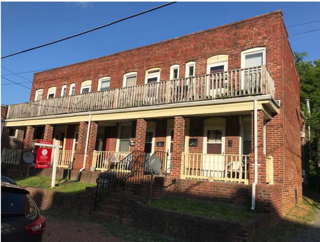
CURRENT PHOTO OF BUILDING - 2020 - FRONT RAILING & DOORS
