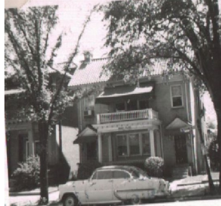
Figure 4. 3105 West Franklin Street, 1950's. Continuous balustrade above the front porch without the center newel post. While blurry, the original porch appears to have fluted Scamozzi columns and dentals.
