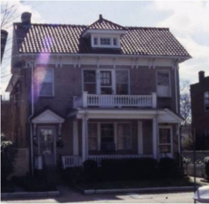
Figure 3. 3105 West Franklin Street, 1998. Balustrade above the front porch. Note, the balustrade did not feature a center newel post.
