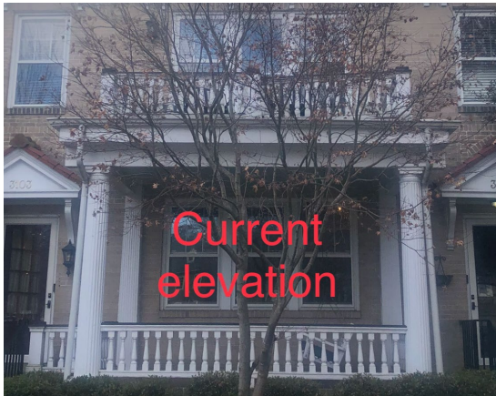
Figure 1. Current façade of 3105 West Franklin Street.
