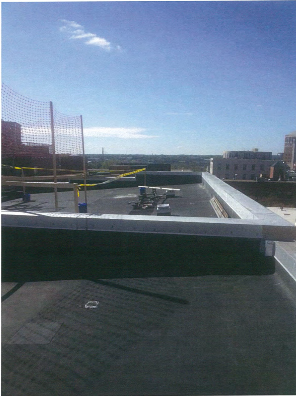
M3. Mockup from roof
