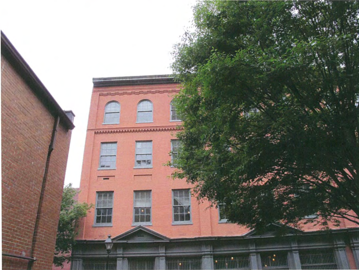
M7. View from parking lot on 13th. Not visible
