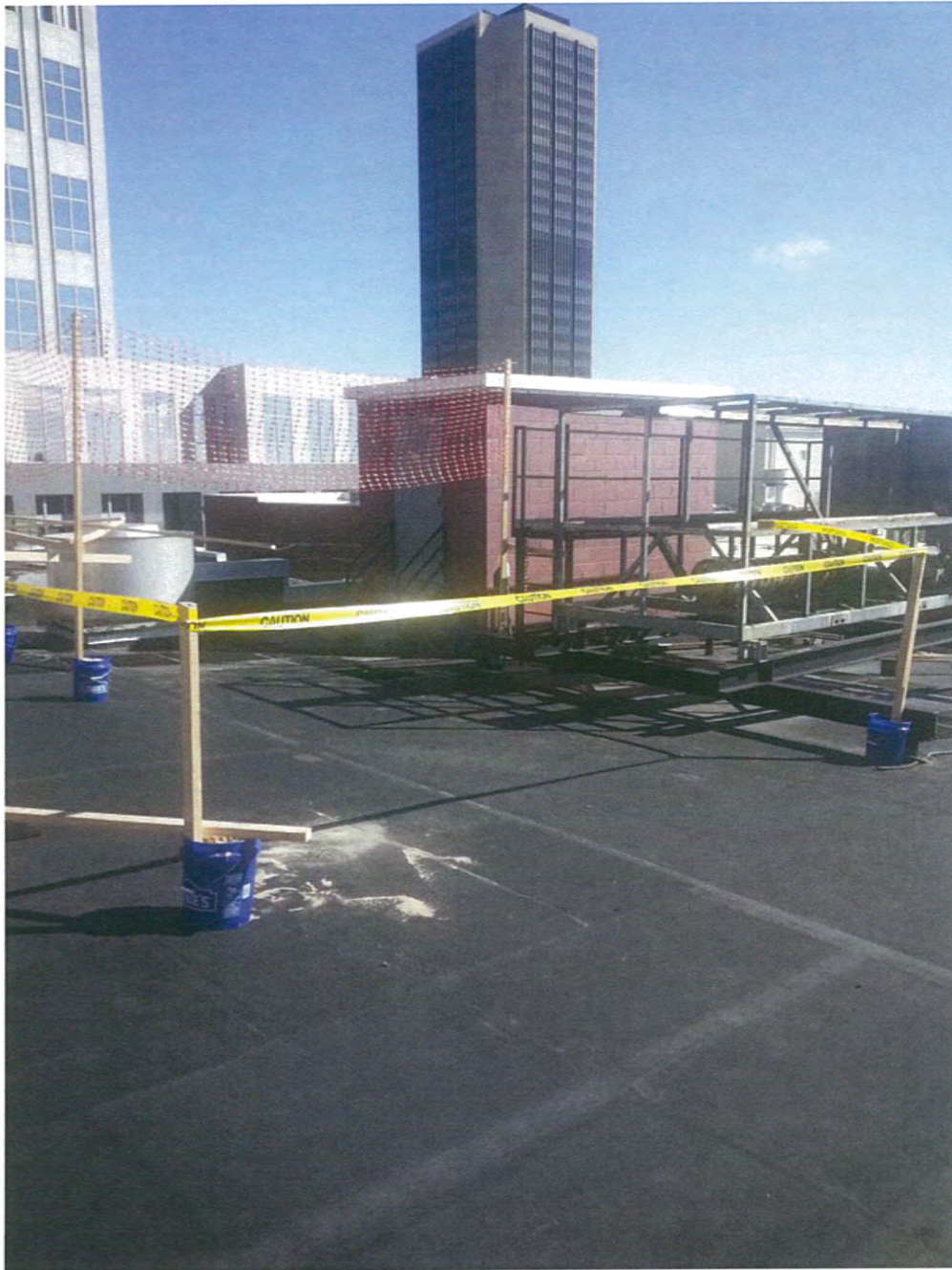
M1. Mockup from roof
