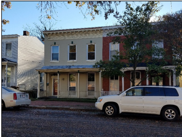
Figure 3. 305 N. 30th Street.
