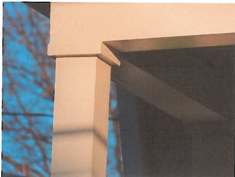
#14 detail view of porch at 815 Jessamine St
