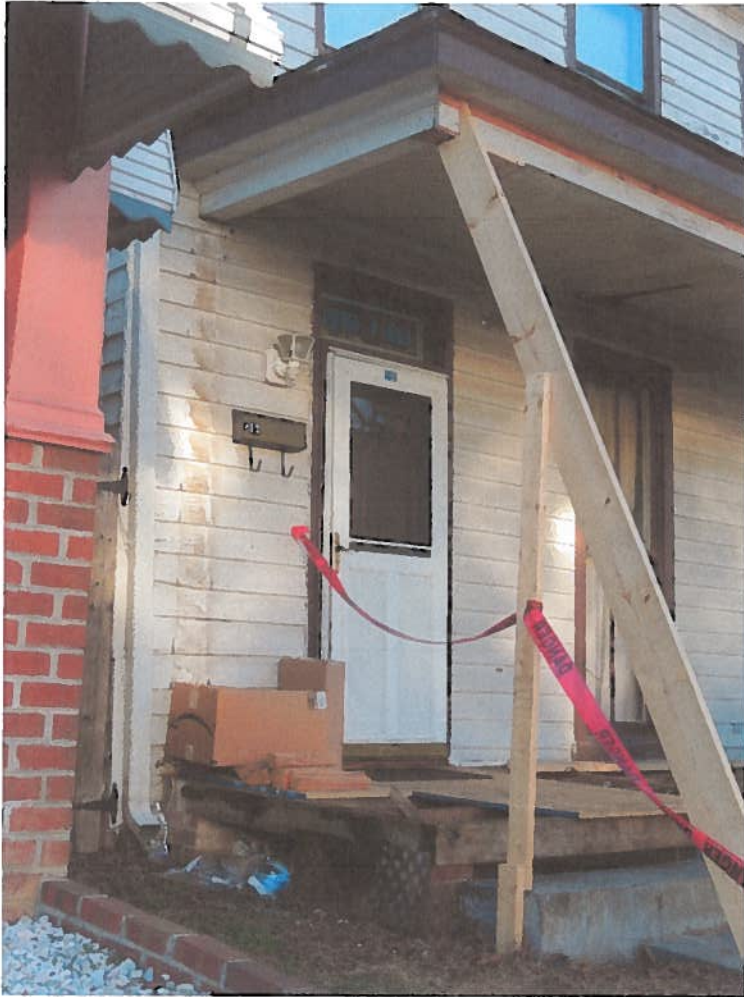
#10 elevation photo of left side of porch
