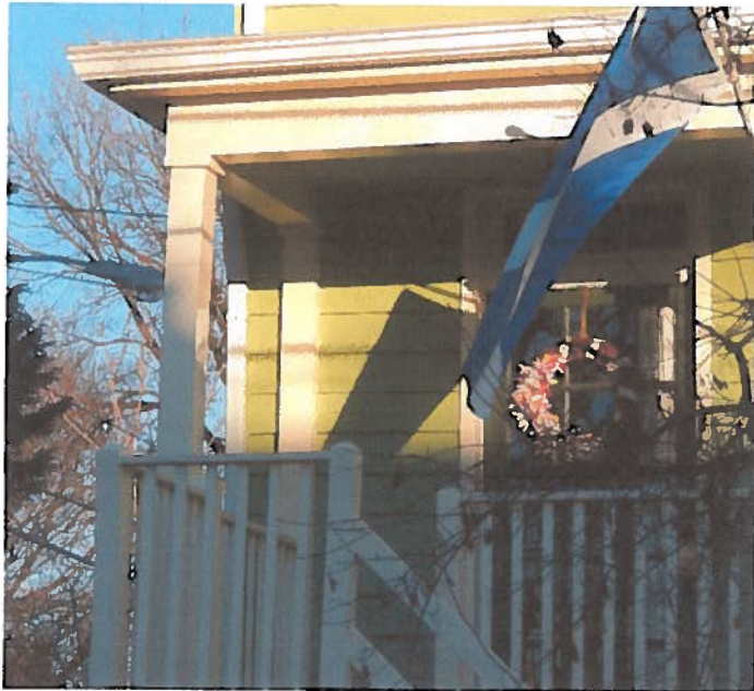
#13 full view of porch at 815 Jessamine
