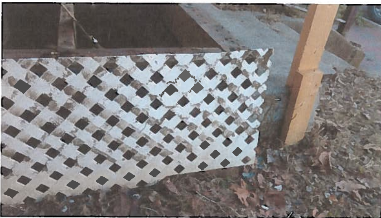
#17 preexisting PVC lattice on the porch skirt
