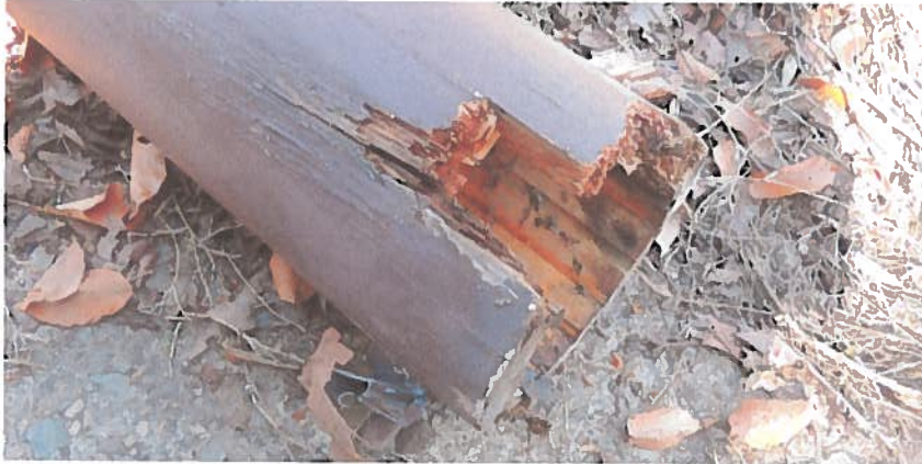
#4 bottom of left corner column
