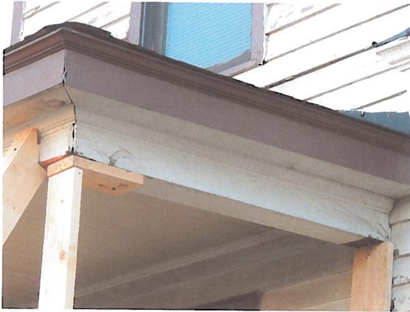
#1 porch roof detail right corner
