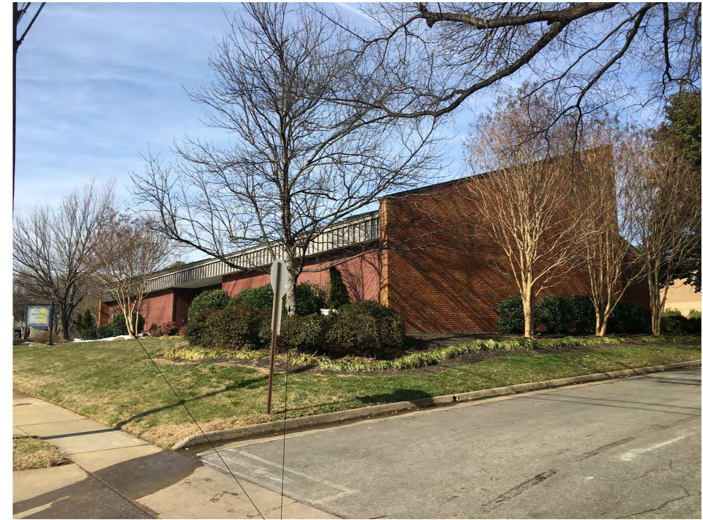
REMOVE TREE DUE TO PROXIMITY TO ROOF AND BUILDING - REMAINDER OF LANDSCAPING TO REMAIN
