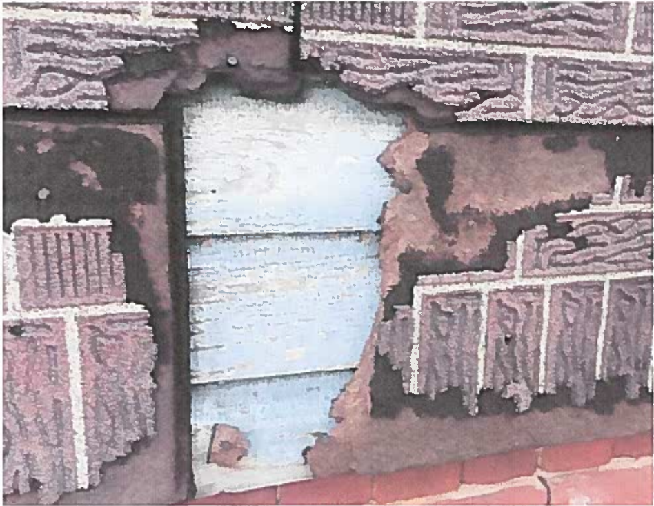
Asphalt Wall Shingle with Original Wood Siding underneath
