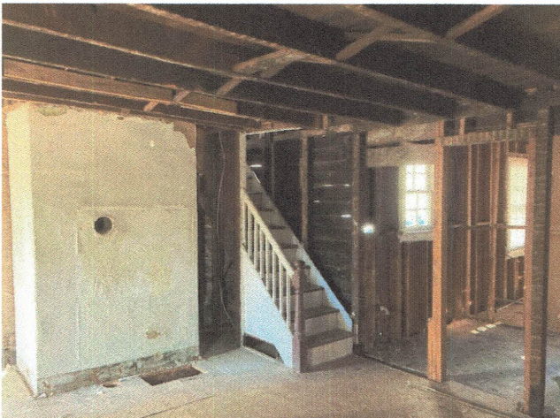
Photo #9 – First Floor Undersize floor joists, long spans
