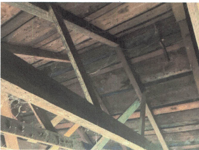
Photo #6 – Strength of roof trusses unknown. Truss spacing 28" – 30". Top chords 4" x 3"
