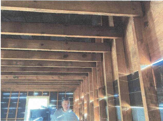
Photo #5 – Improper ceiling joist connections to studs. Above these, Roof Rafters 2 x 6 at 36" oc
