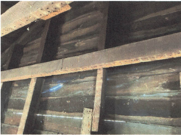
Photo #8 – Discontinuous studs.
