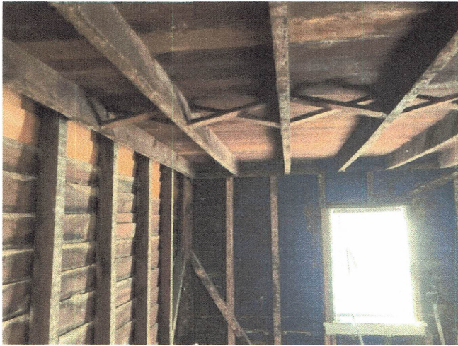
Photo #4 – Undersized floor joists. No sheathing or moisture barrier on exterior walls.
