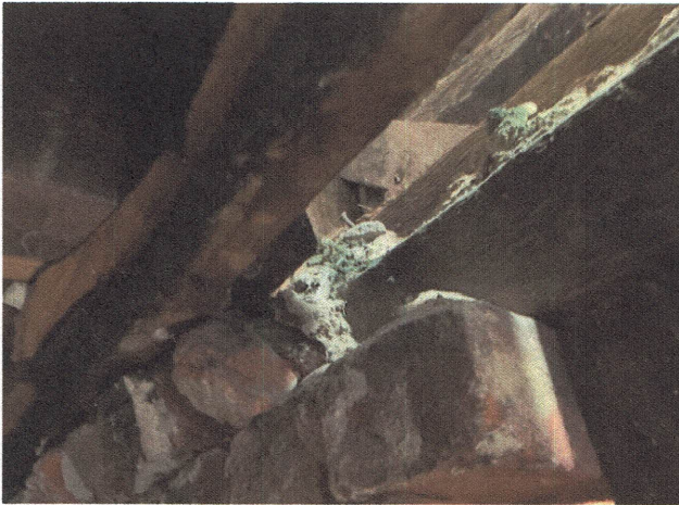
Photo #2 – Crumbling Foundation. Brick missing.
