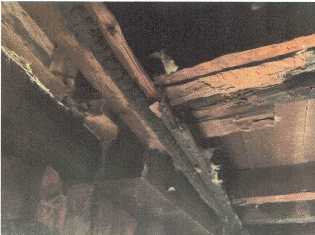
Photo #3 – Rotten, charred and undersized beams in basement.
