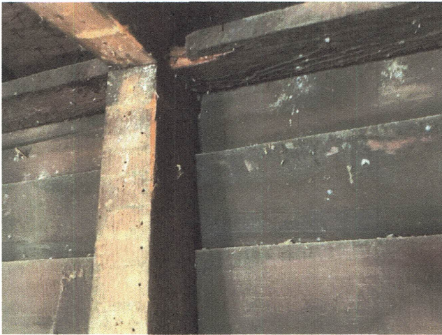
Photo #7 – Rotten wood single top plates, Fire Charr.
