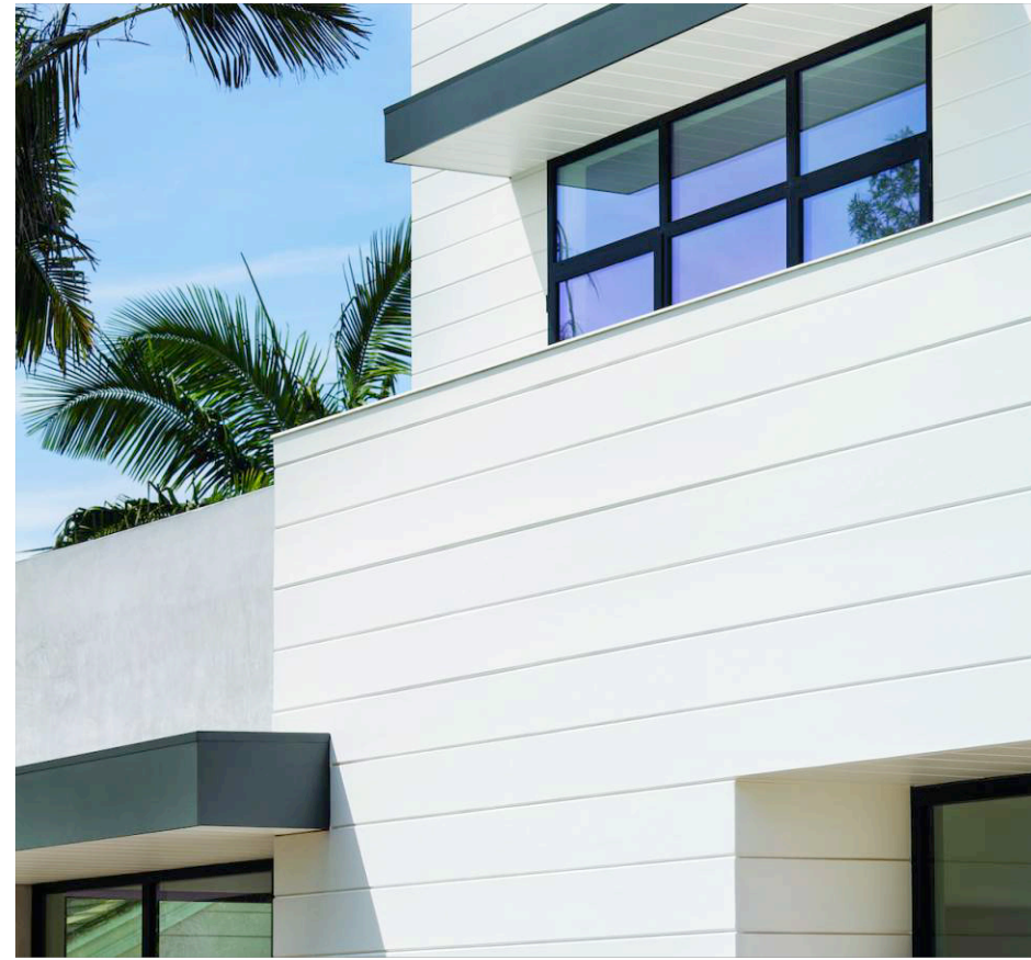
3RD FLOOR CLADDING
