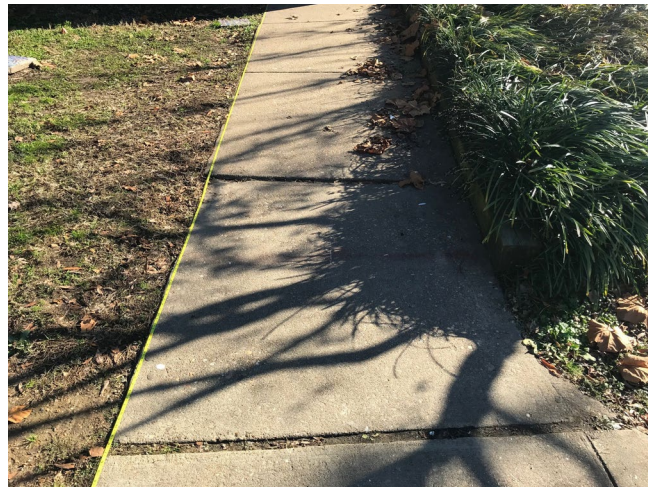
Sidewalk to community center entrance
