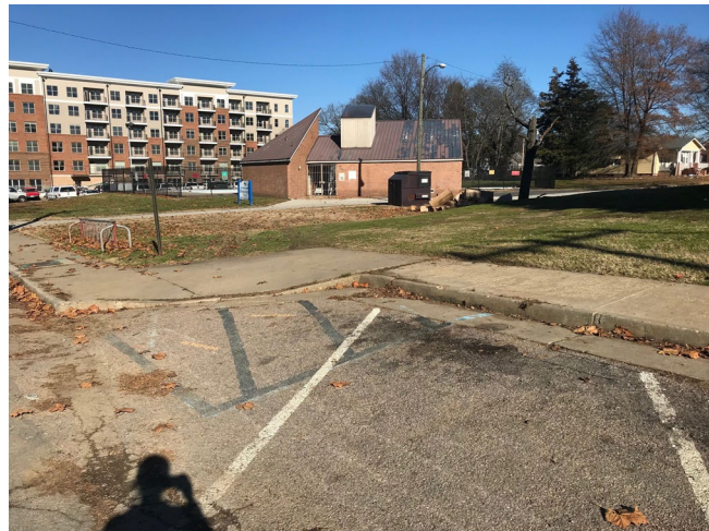
Curb ramp at community center entrance.
