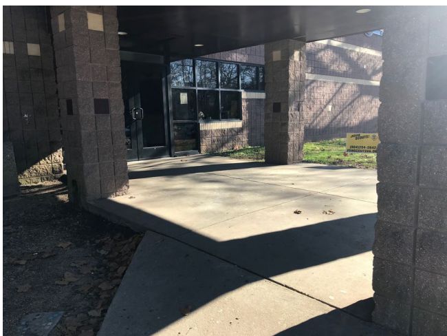
Detail view of community center covered entry.
