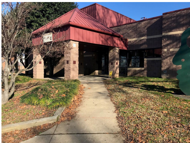
Secondary sidewalk at community center entrance to remain.
