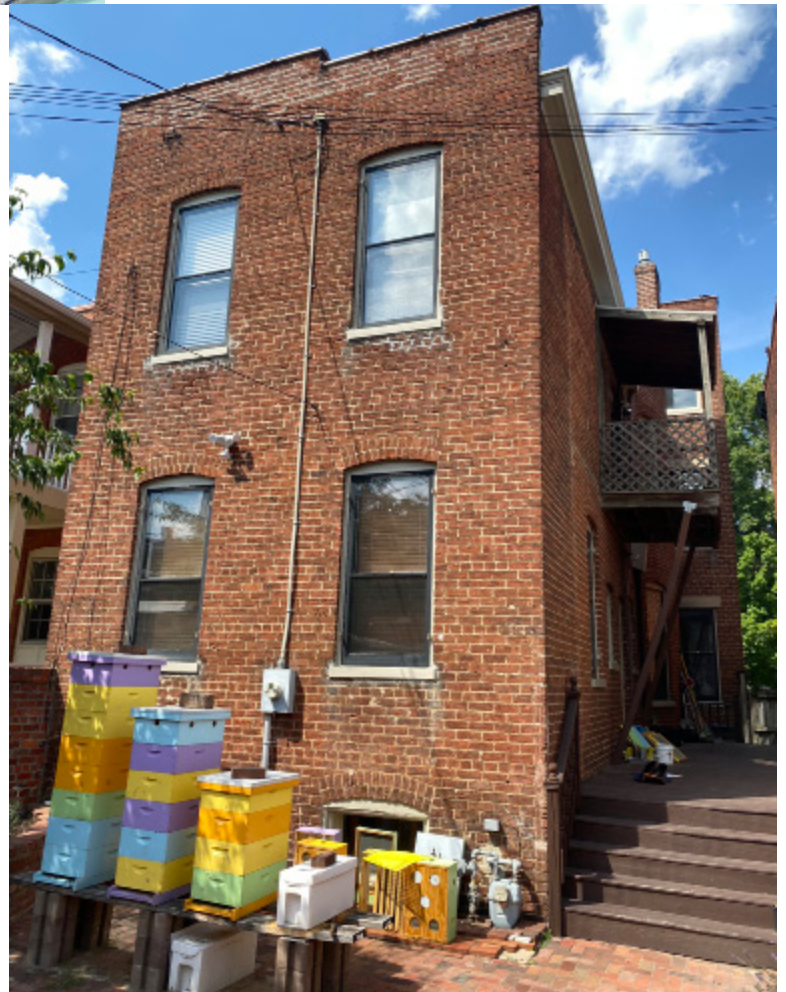
REAR OF EXISTING HOUSE FACING ALLEY
