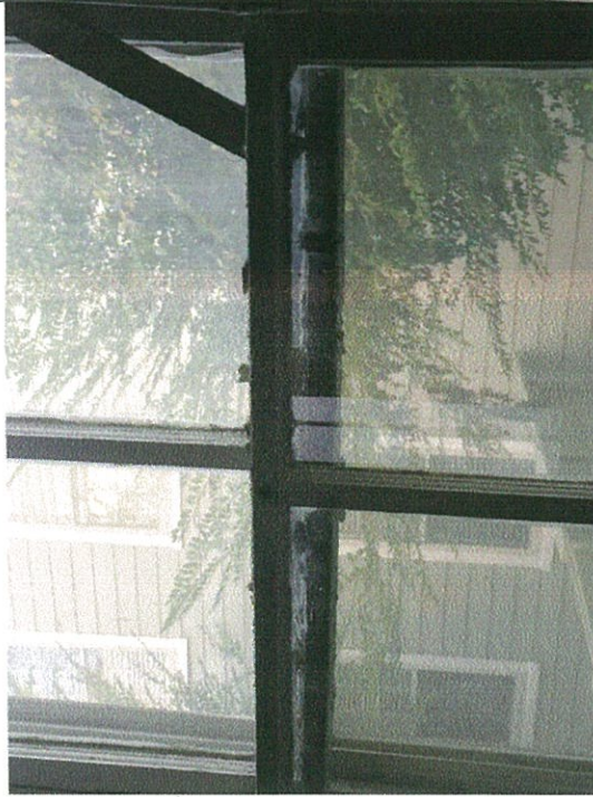
#1 window is inoperable and is being held together by a nailed piece of wood
