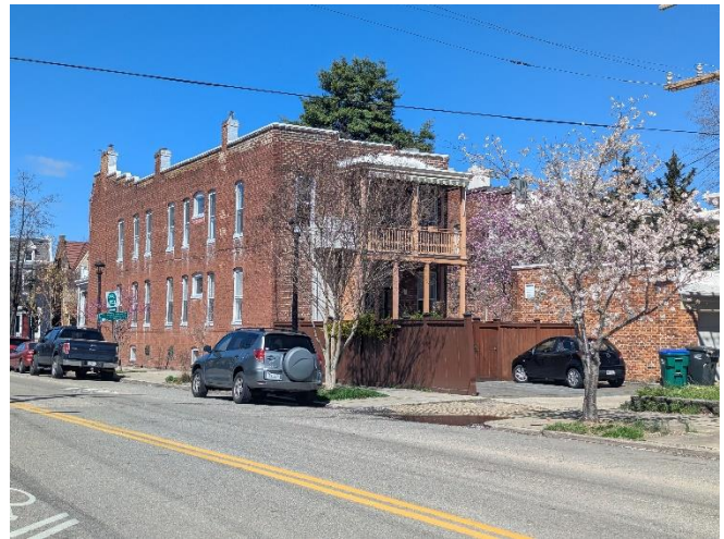
Figure 2: Site photo showing the prominence of the lot on Floyd Avenue, and the high visibility of its rear section.
