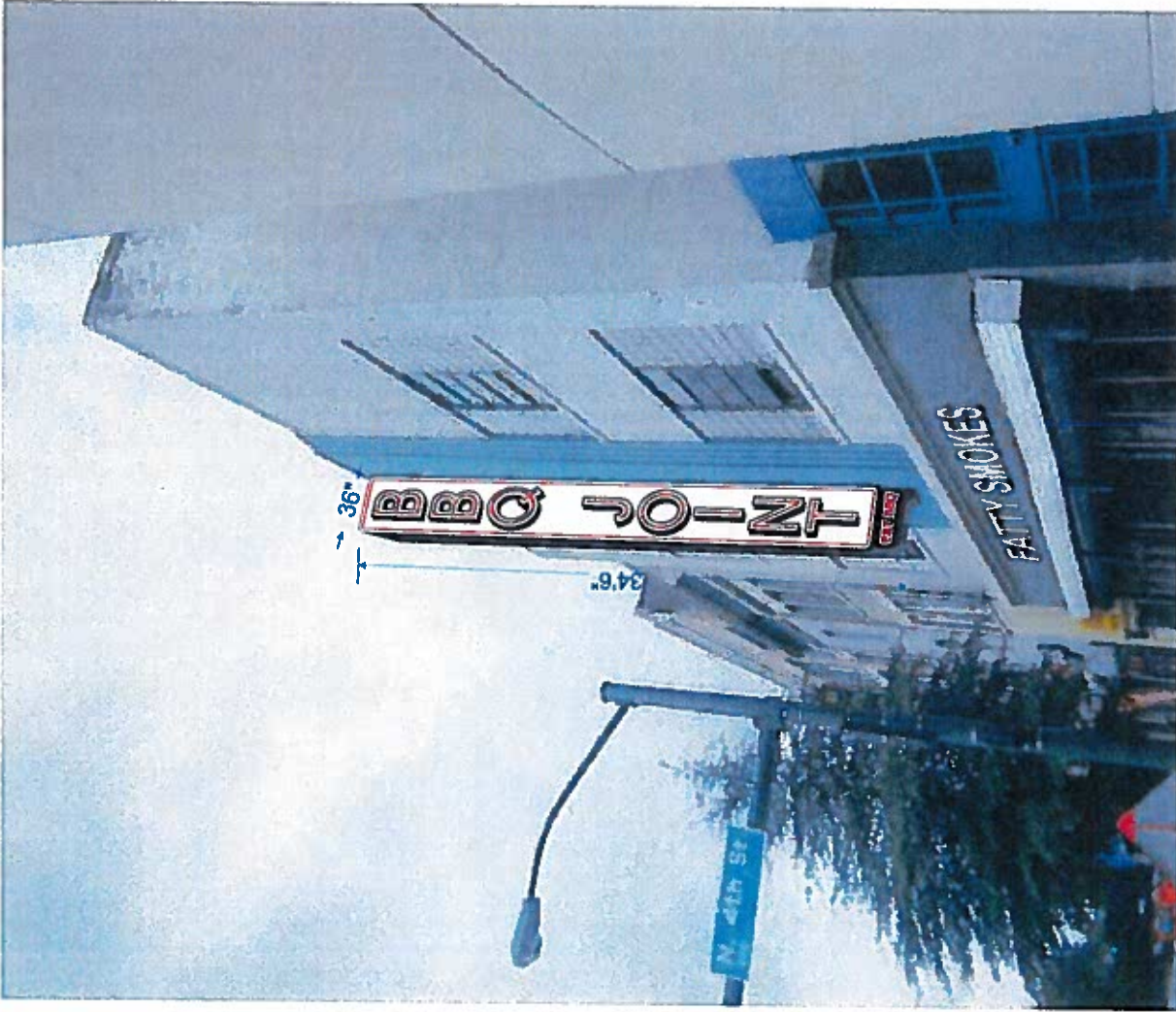
Channel letters red neon sign. Clear plexiglass faces, red neon lighting, black trim caps, black returns. Sizes and colors as depicted on the drawing.
