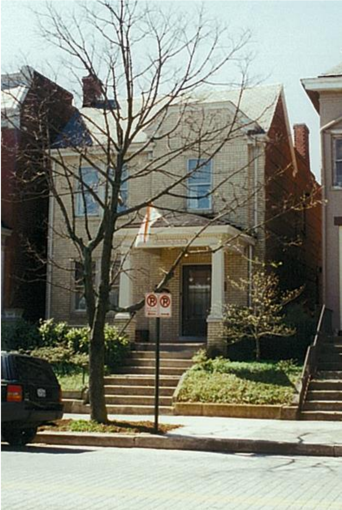
Photograph of 2241 W. Grace Street from 1996 Photographic Survey.
