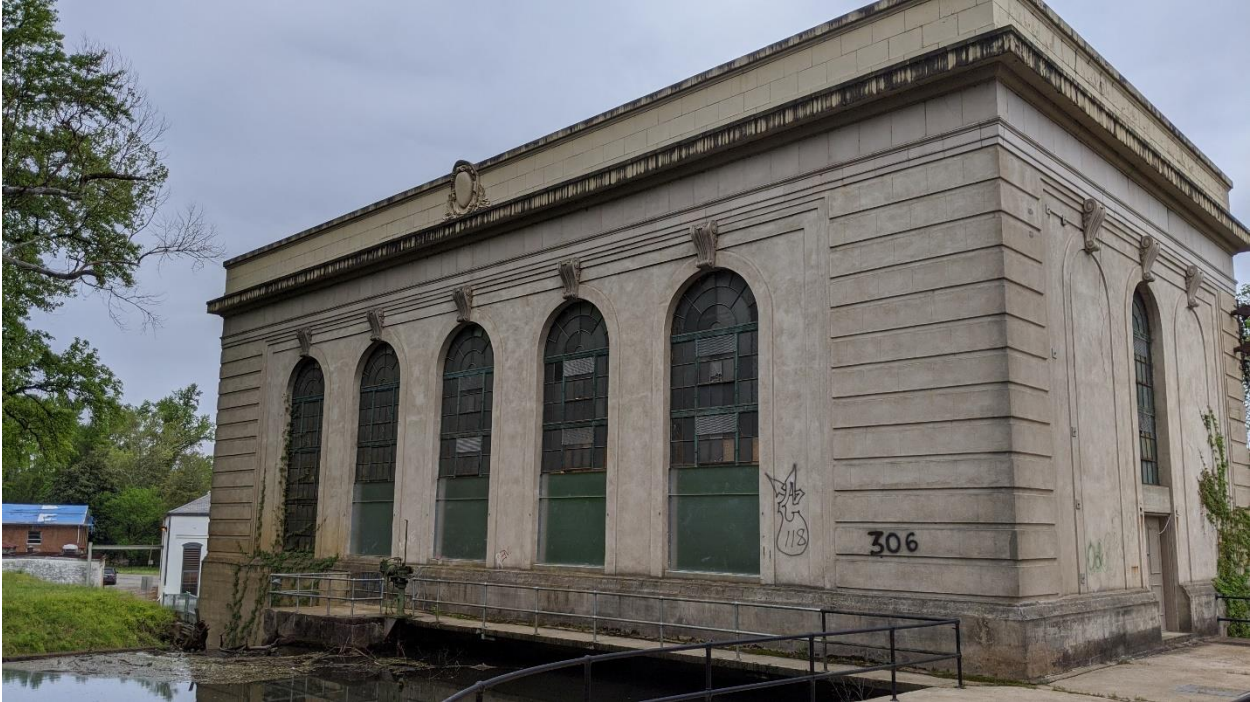
North façade showing the existing blank off panels at the bottom of the windows.
