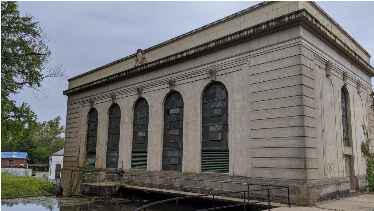
The North façade as it could look with the new louvers installed.
