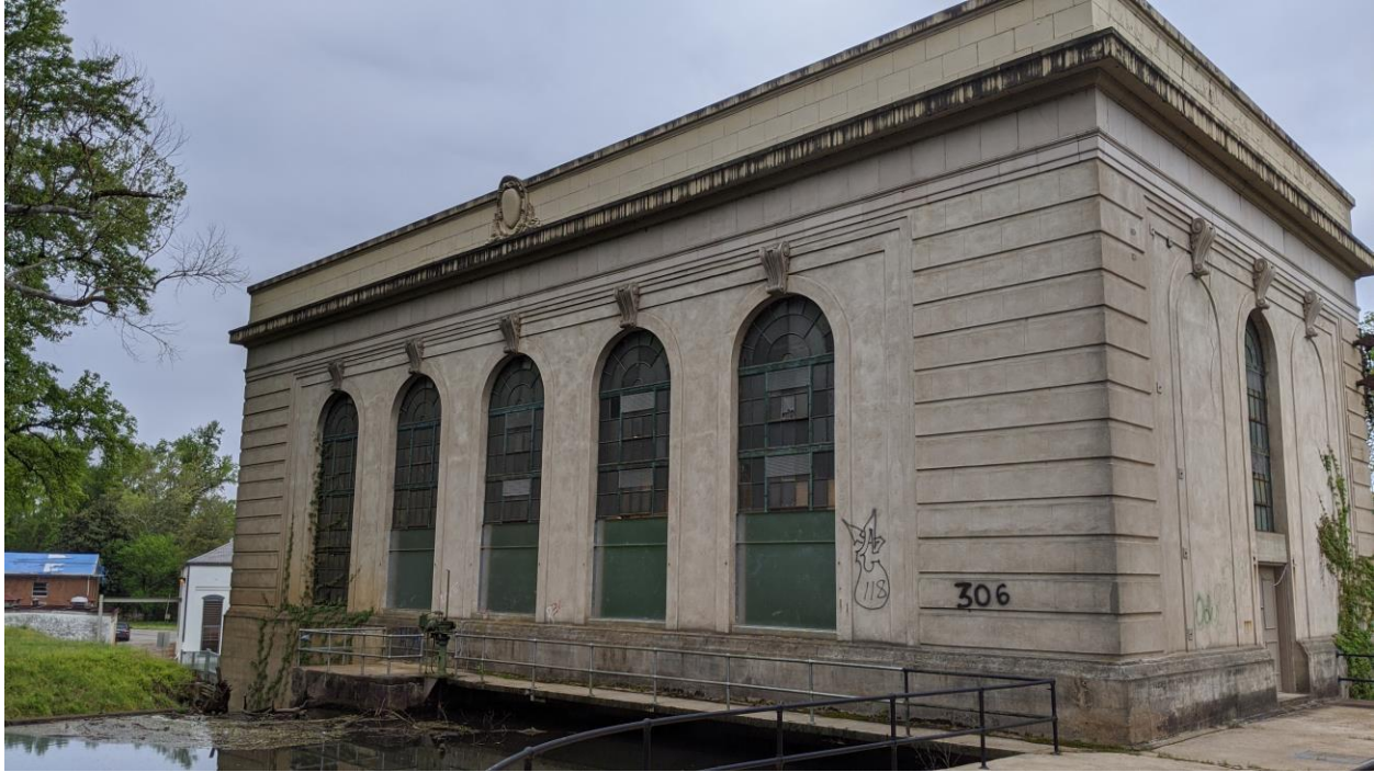
North façade existing condition
