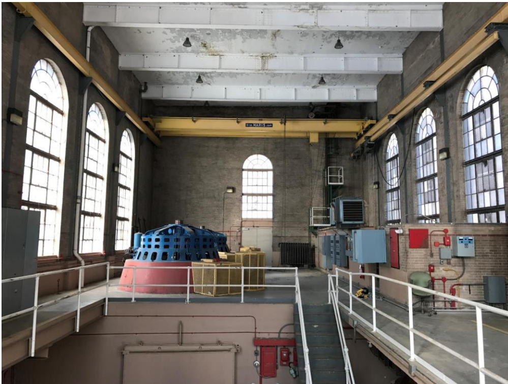
Main floor looking west.
