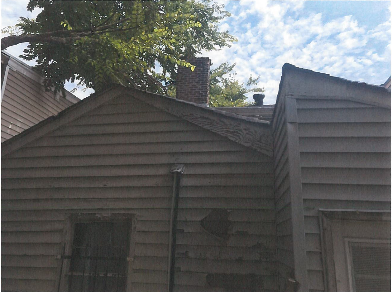
Rear Exterior showing existing asphalt shingles
