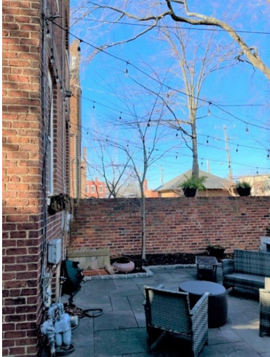
Figure 2. Rear brick wall and site of new screened-in porch
