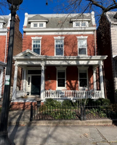
Figure 1. Front facade, 2606 W. Grace Street
