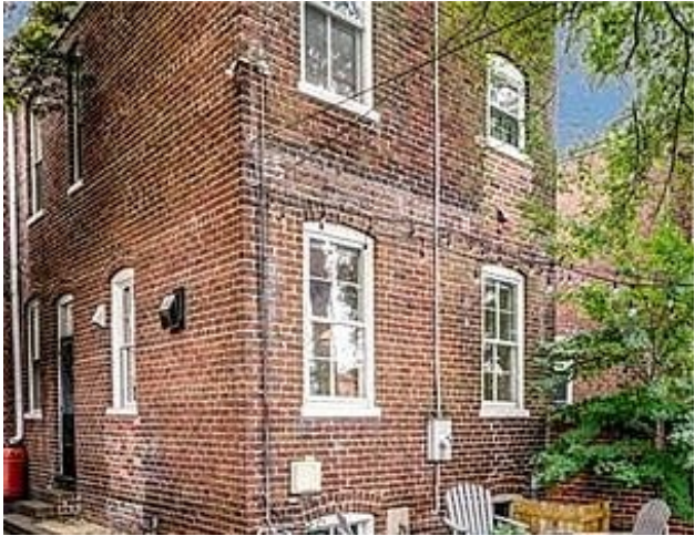
Figure 4. Rear window details. Minimally visible from alley. (Zillow.com)
