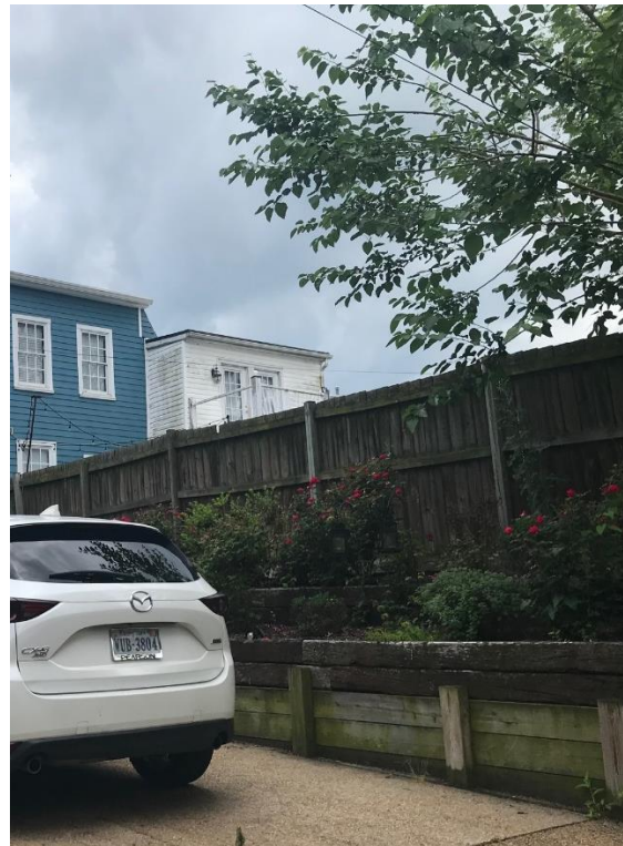
Figure 4. Rear deck, viewed from alley
