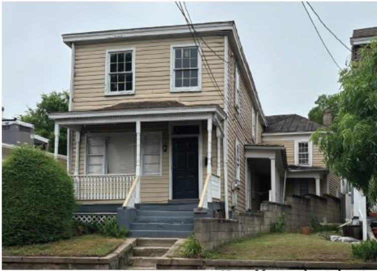
View of front and east elevations Note: The roof structure, frieze beam, fascia, dental molding, crown, brick masonry piers, appear to be original and will be retained and restored. The remainder of the porch will be replaced as shown in the attached documents..
