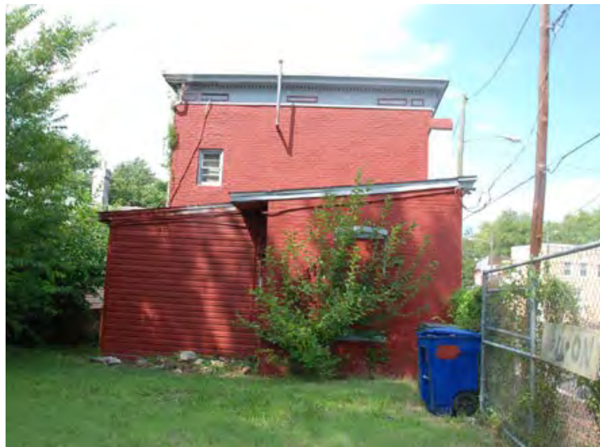
View at South Elevation showing brick 1-story section along N 21st Street and adjacent framed section. Framed section is proposed to be demolished with new addition extending from its location.
