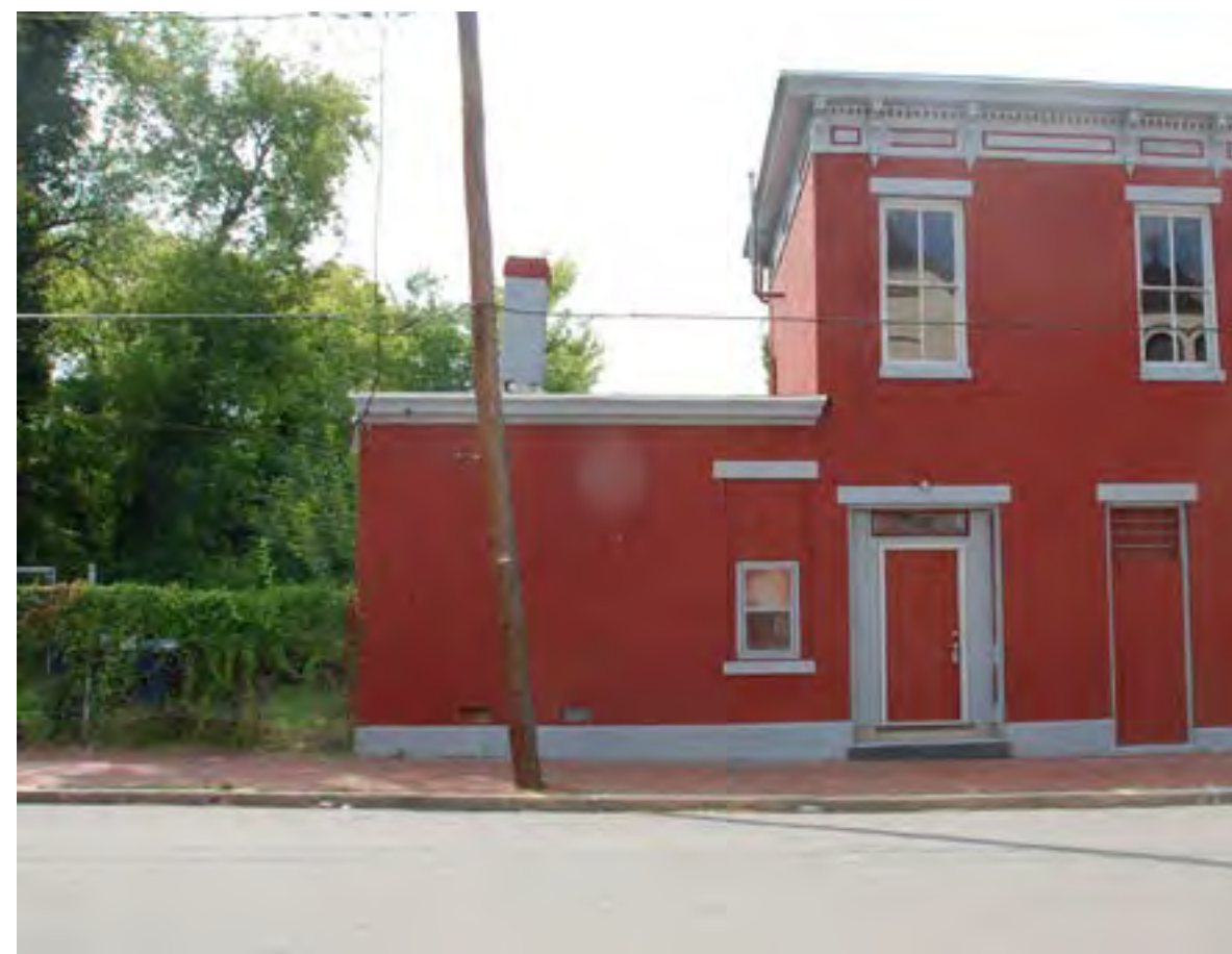
South End of Historic Structure at 1-story masonry section - proposed addition is positioned behind this area in the rear yard which extends to Burton Street (alley)
