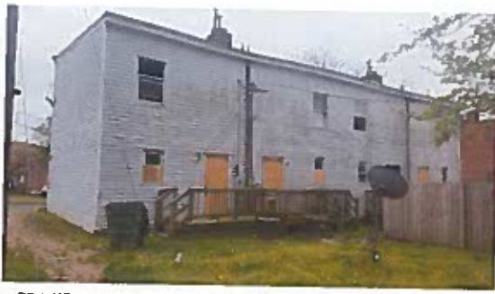
FIG 4 - VIEW OF NORTHREAR FACADE
