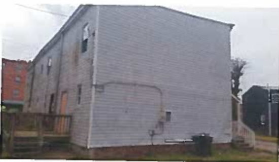
FIG 3 - VIEW OF WEST FACADE
