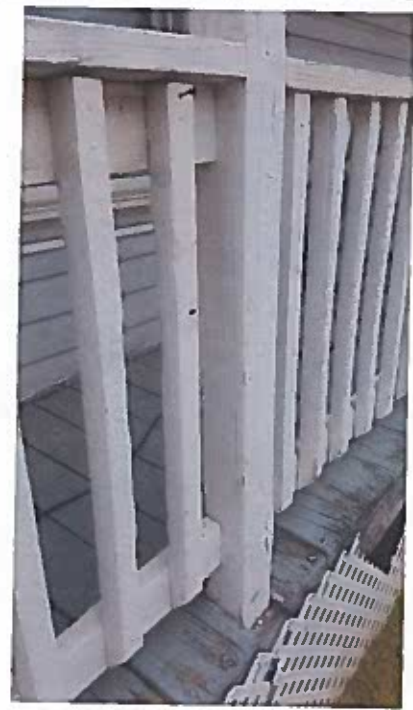
FIG 7 - VIEW OF FRONT PORCH RAILINGS, 2X4 RAILS WITH 2X2 PICKETS
