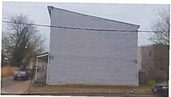
FIG 5 - VIEW OF EAST FACADE
