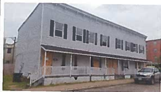
FIG 2 - VIEW OF SOUTHFRONT FACADE
