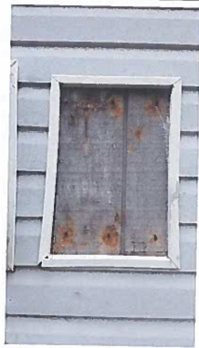
FIG 6 - VIEW OF VINYL SIDING AND T1-11 PANELING AT WEST FACADE
