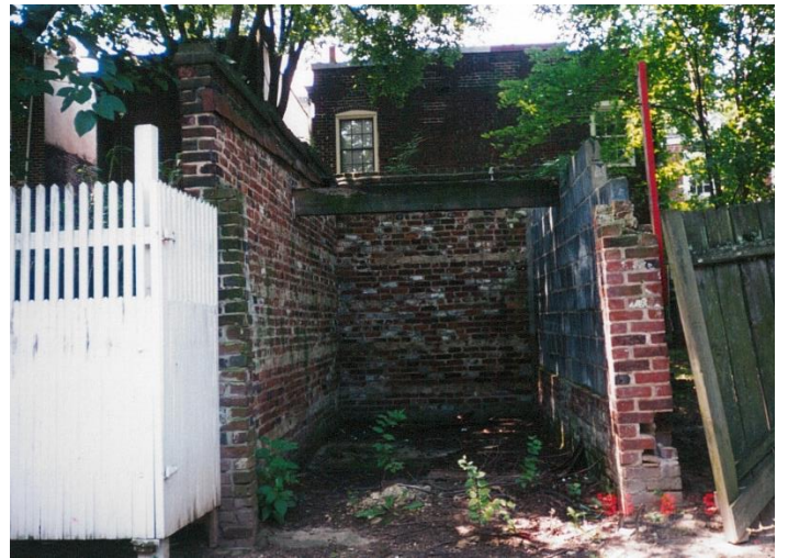
Figure 4. Garage prior to rehabilitation, 1996
