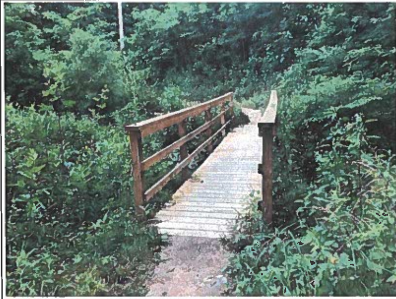
20. Bridge Facing West (262°) Location from Geneq iSXBlueII 20200618_RIC_4530_CityofRichmond_LewisGLarusPark_020.jpg
