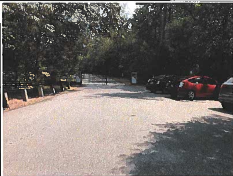
1. Parking lot at Sabot School (Wukong's Path) Facing North (18°) Location from Geneq iSXBlell 20200618_RIC_4530_CityofRichmond_LewisGLar usPark_001.jpg
