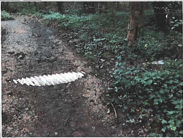
19. Culvert Facing Northeast (39°) Location from Geneq iSXBlueII 20200618_RIC_4530_CityofRichmond_LewisGLarusPark_019.jpg
