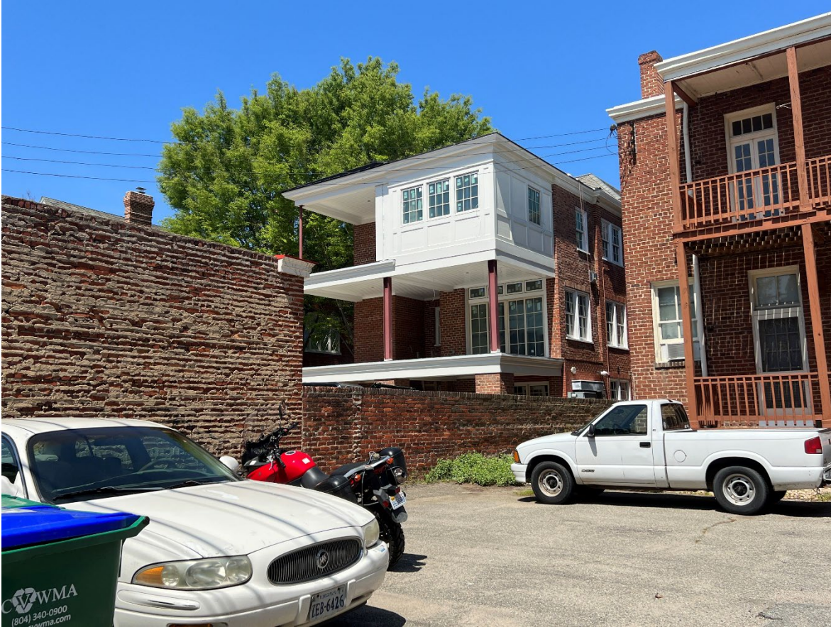
Figure 1. Location of rear brick wall that will be increased in height. New free-standing chimney will project above this portion of the wall.
