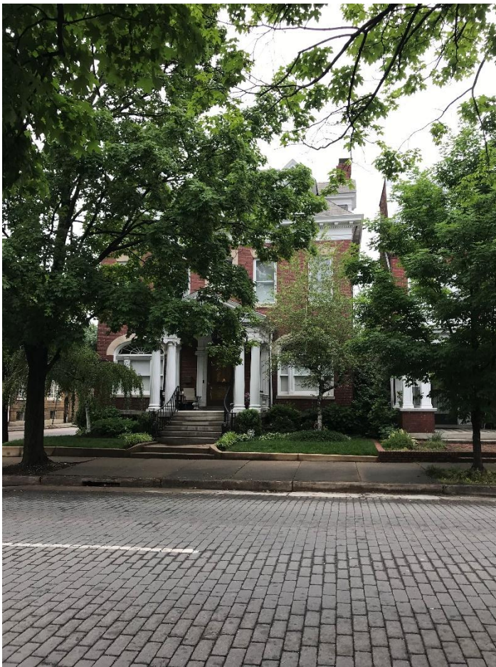
Figure 1. 2516 Monument Ave, facade
