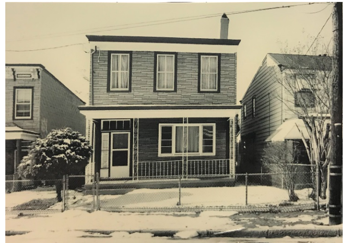
Figure 4. 706 North 21st Street, ca. 1993.
