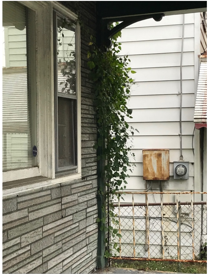
Figure 6. 706 North 21st Street, column detail.
