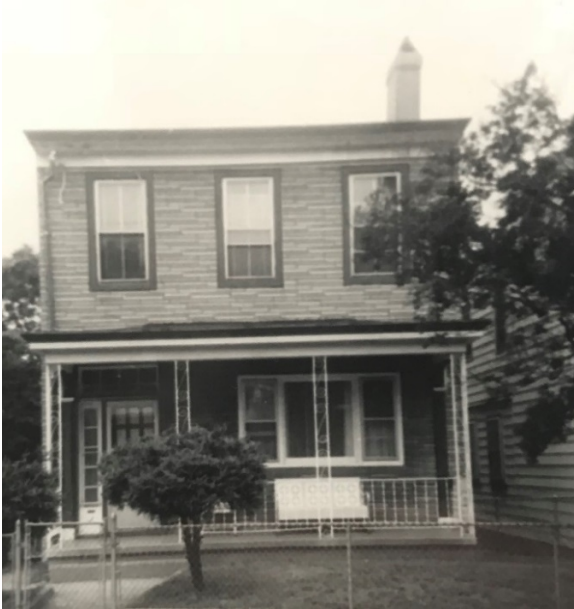
Figure 3. 706 North 21st Street, ca. 1977.
