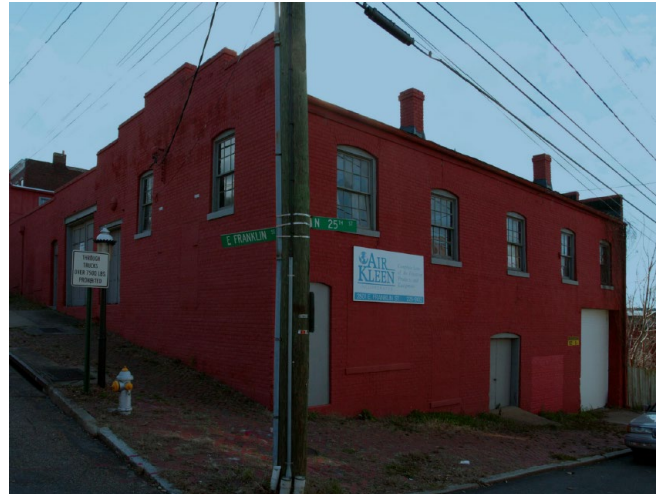
Figure 2. 2501 E. Franklin, date unknown, photo provided by applicant showing past condition of building.
