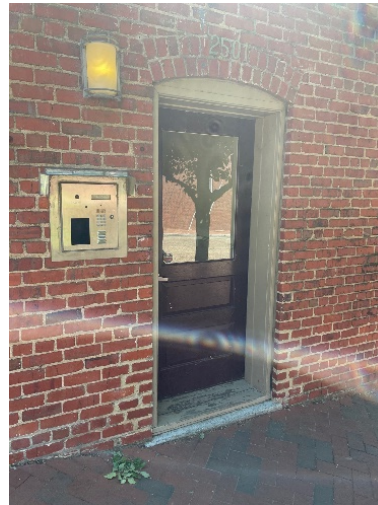
Figure 4. 2501 E. Franklin, existing conditions, other door on subject building.
