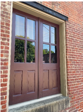
Figure 5. 2501 E. Franklin, existing conditions, other set of doors on subject building.
