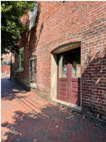
Figure 3. 2501 E. Franklin, existing subject doors and single-pane windows
