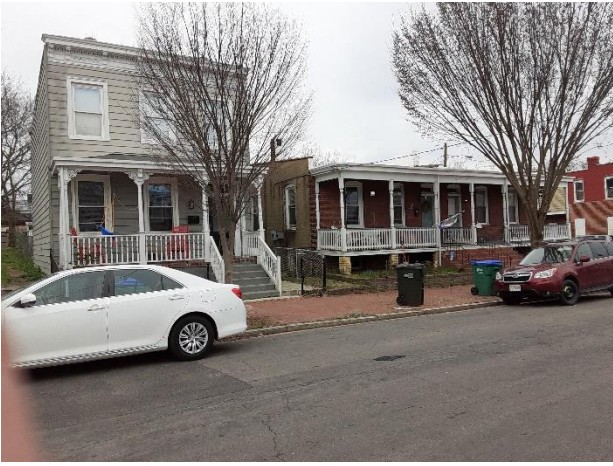
Figure 7. 901-905 N. 24th Street.
