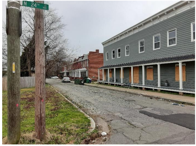
Figure 8. 2300 block of Burton Street.
