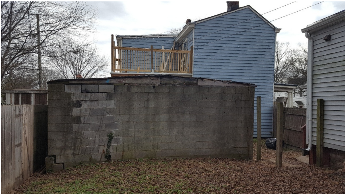
PHOTO 10 GARAGE WEST / SIDE ELEVATION (FACING CHIMBORAZO BLVD.)
