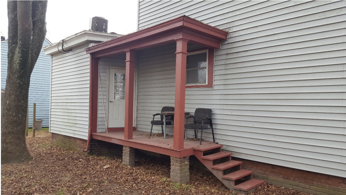
PHOTO 5 NORTH / SIDE PORCH
