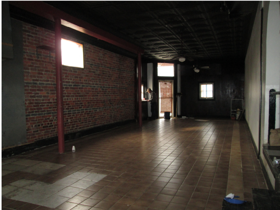
PHOTO 12 MAIN INTERIOR SPACE LOOKING TOWARDS FRONT
