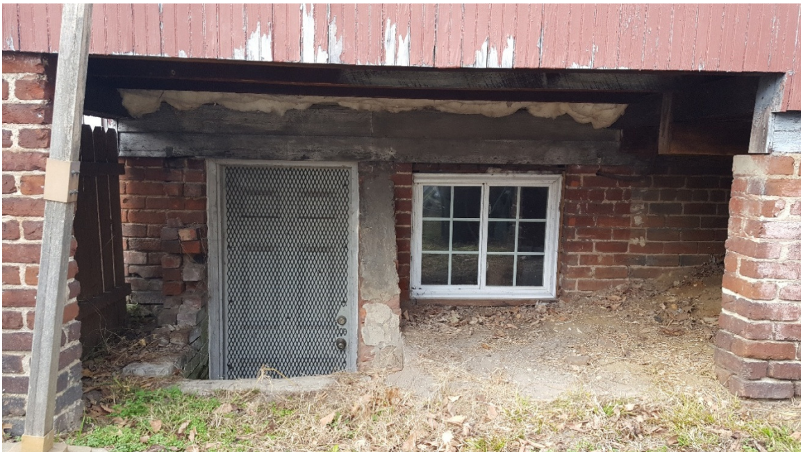
IMAGE 4 BASEMENT ENTRANCE UNDER REAR PORCH
