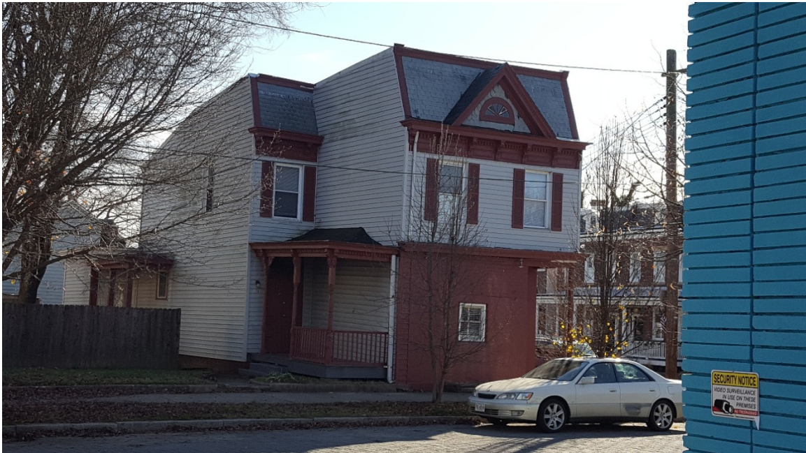
PHOTO 2 WEST / FRONT – NORTH / SIDE ELEVATION
