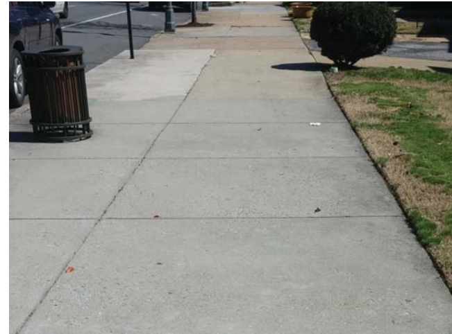
BRUSHED CONCRETE: EXISTING SIDEWALK, REPAIRED AS NEEDED, MARKS THE PATH FOR PEDESTRIANS. CONCRETE CLEARLY DEFINES DRIVEWAY ENTRANCES WHERE IT CROSSES THE TIGHTER GRIDDED SCORING PATTERN.
