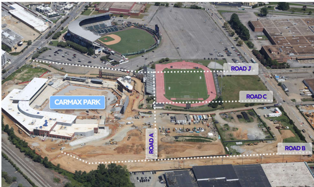
Exhibit B: Aerial image taken August 22, 2025 shows the alignment of future roads on the current site (Source: Diamond District Partners, LLC)
