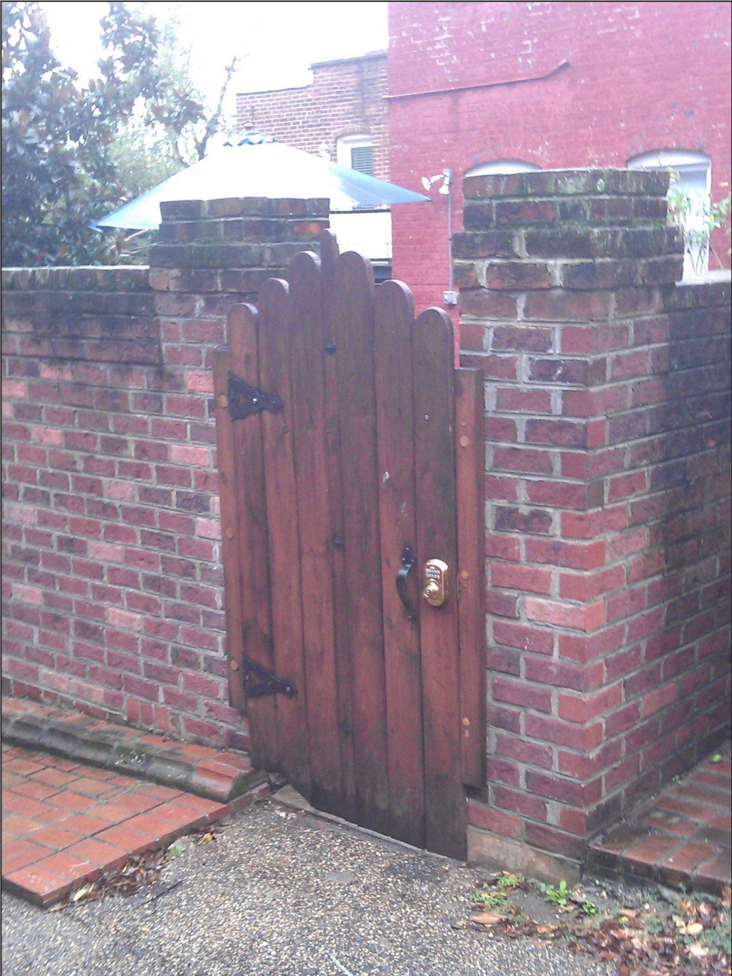
Example of proposed gate, located in the N. 25th-26th Streets' alley, between E. Broad St and E. Grace St.
