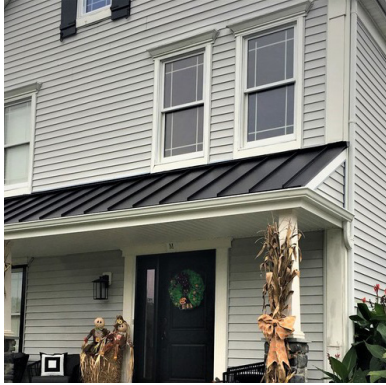
Standing Seam Metal Roof
